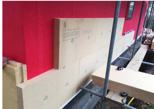
Breathable external insulation skin removes thermal bridges
