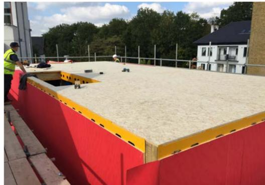
OSB fixed to floor joists
