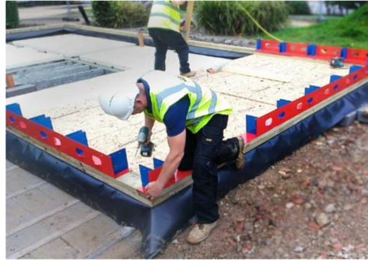
Factory laser cut steel structural ring beam
